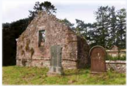
St. Mungo's Church
